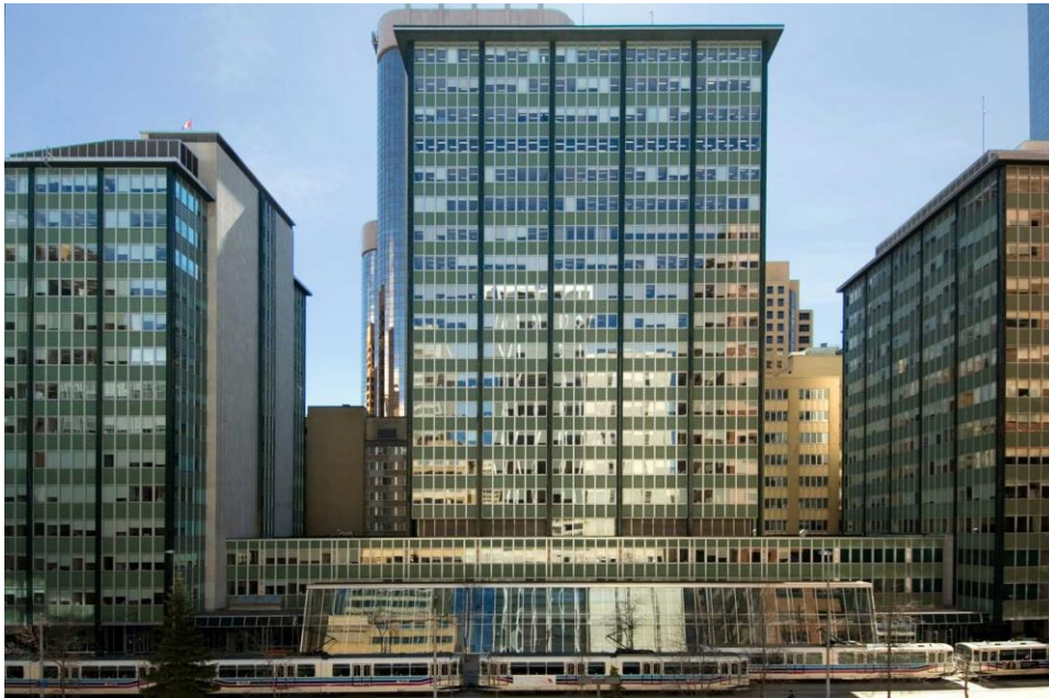
(The Elveden Centre at 727 7th Ave SW in Calgary, Alberta. Source : Photo by Chuck Szmurlo taken April 13,200. ( Lien ))
